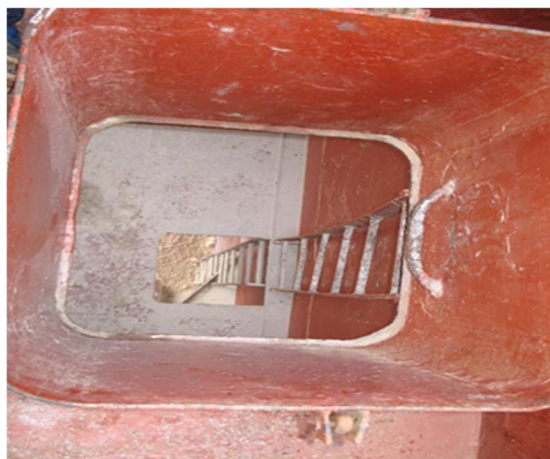
Fig. 3 View from the entrance hatch to the vertical ladder
