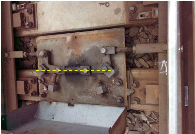
Fig. 2. Switch №20 spring rocker arm, set in unregulated (equilibrium) position
